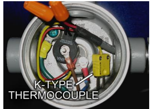
Figure 12.7 Heater Thermocouple
