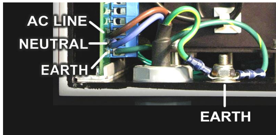
Figure 3.19 Transmitter AC Connections
